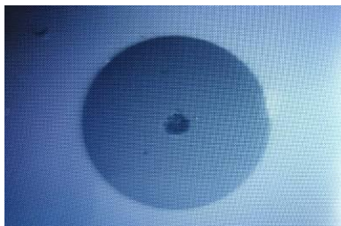
Damaged: Replacement required
